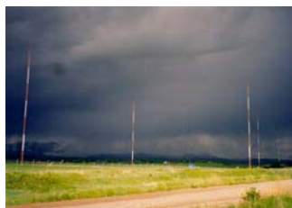
Operating at 60 kHz, antennas for WWVB are huge, measuring 100s of meters.
