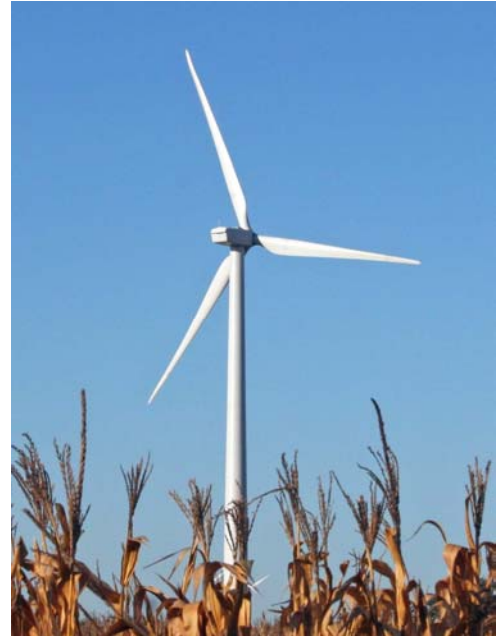
The diameter of a single wind turbine prop can equal the size of a football field. The speed at the prop tips can reach 120 MPH.
